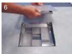
6 Remove the frame and trap by loosening the four corner
