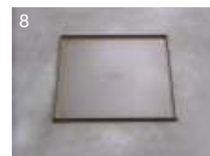
8 Finished installation without the carpet
